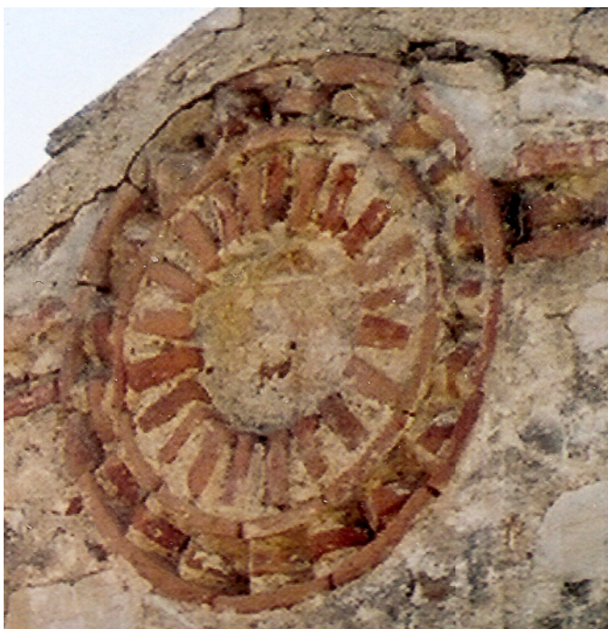
Fig. 60. Myrtia, Myrtia Monastery, katholikon, E façade. Detail of masonry.
